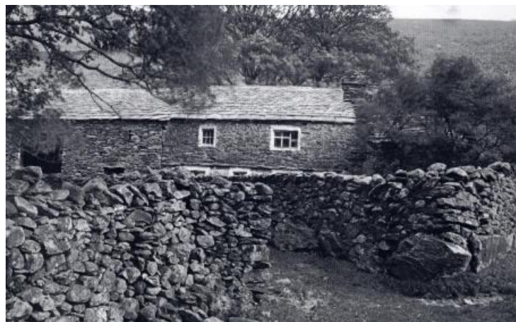
Braken Howe farm as it once was, this is one of the first ruins to show when the water is low
